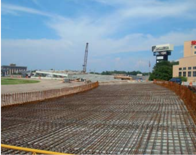
Set slab reinforcement steel
